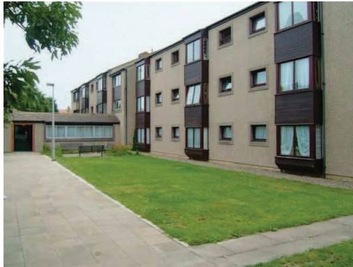
Council owned housing at Kingsway Court, Heysham
