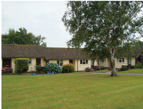
Lancaster City Council owned accommodation for older people at Vale Estate, Lancaster
